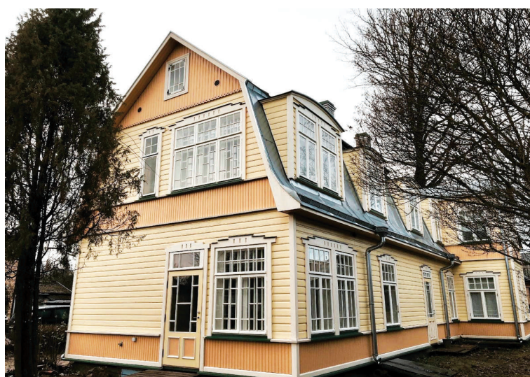
House after renovation. Photo: J.Laineste
