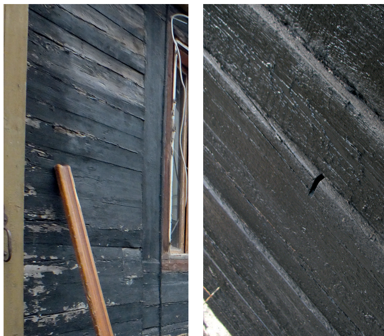
The walls before restoration.
