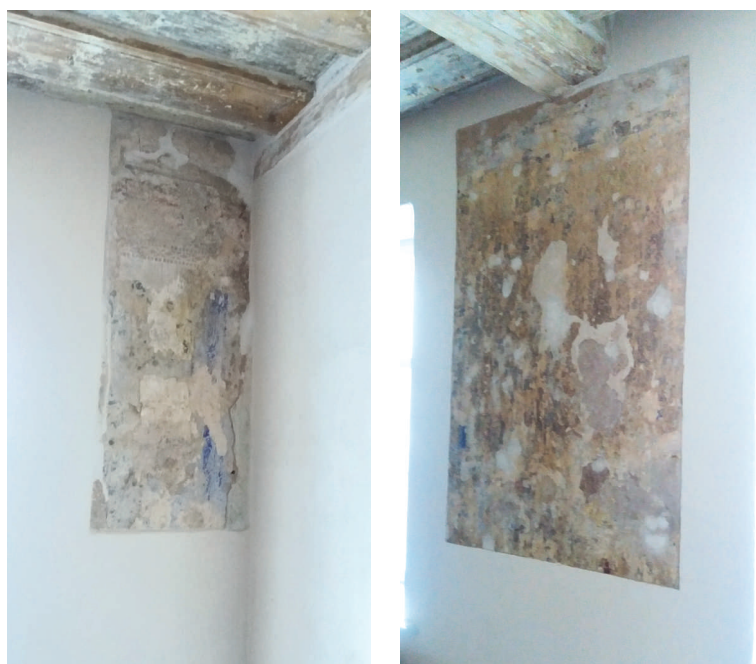
The preserved current and newly formed lime mortar plastering
