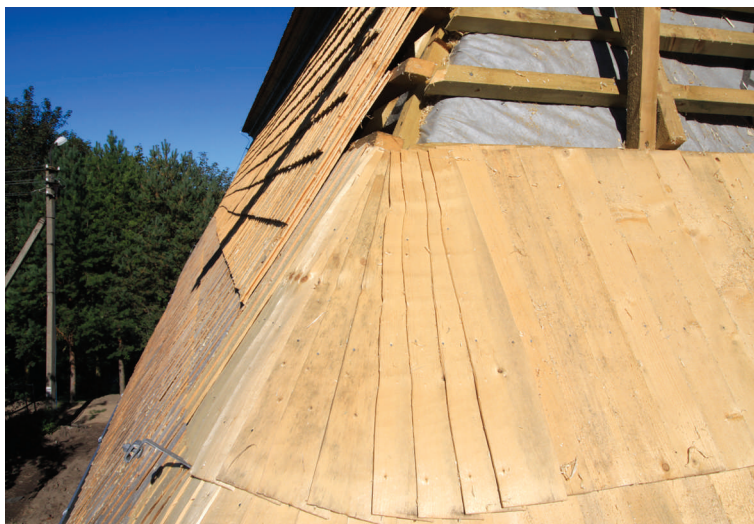
Spruce shingle roof covering 2017. (photo M. Veliulis)
