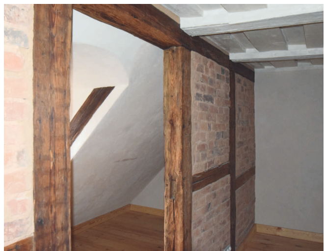
After the rebuilding renovation. The cold porches partly incorporated with the heated premises – with some openings in the filled framework walls, in order to ensure more lighting from the built-in roof parts
