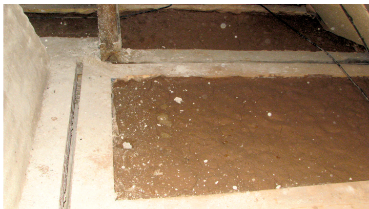
The removed and repeatedly laid clay covering
