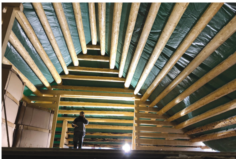
Inside the attic before the ceiling is put on top of the logs
