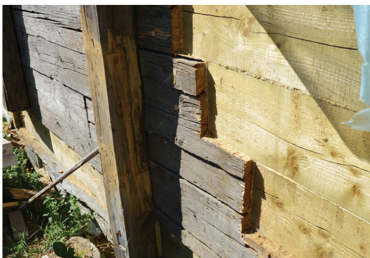
Wall insulation and boarding of the synagogue 2017 (photo M. Veliulis)
