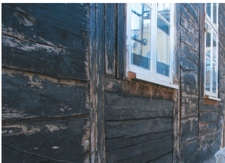
The window block application in various material walls with the supplements – flax tows 13
