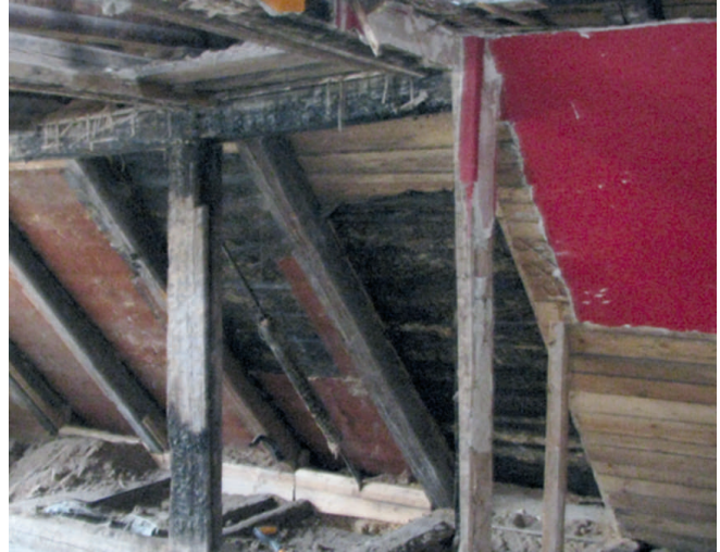
The renovation processes. The cold porches and their construction
