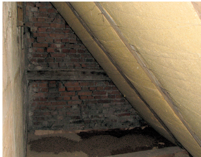
The insulation of roof board with wood fiber boards
