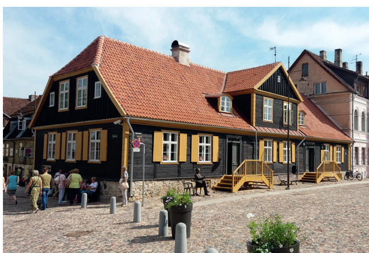
The building in the beginning of the 20th century – with wall rendering on the wooden log house walls 3 and the building after the renovation – in 2016
